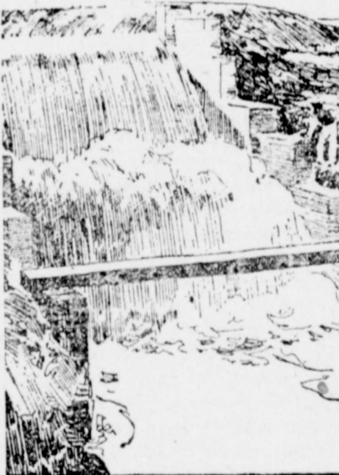
A Drop Just After the Water Leaves the Gates of the Lake on the Way to the Irrigation Ditches.
