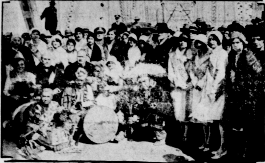
Governor Arthur Weaver of Nebraska (left) and Governor John Hammill of Iowa (right) are shown seated in the group which assisted in the dedication of a new bridge over the Missouri river at Nebraska City, Neb. In front of them, at left, in Indian costume, is William Hale Waubonsie, descendant of the Indian chief Waubonsie, for whom the bridge is named.
