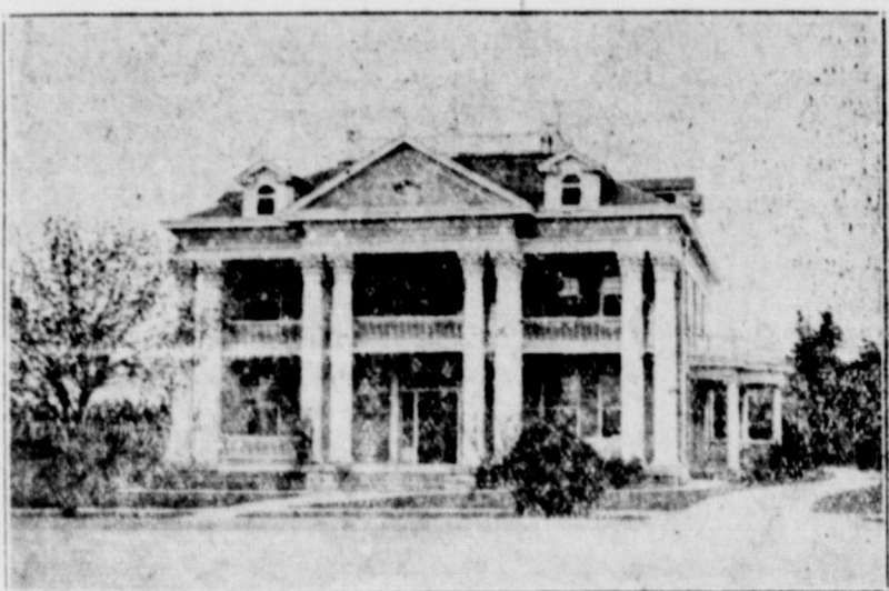
The Home—Corner of Broadway and Park Avenue
