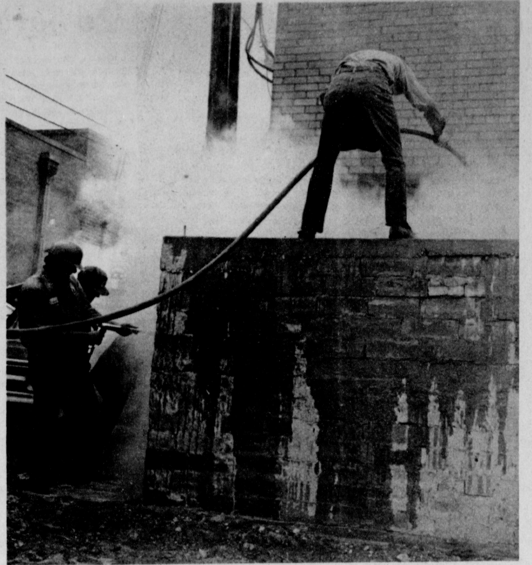
SMOKE GETS IN YOUR EYE . . . Lots of smoke, but little fire was what firemen found when they answered a call to White's Cashway Grocery Wednesday at noon. A fire had started in a box storage area adjacent to the store. No damage was reported to the store or its contents.
