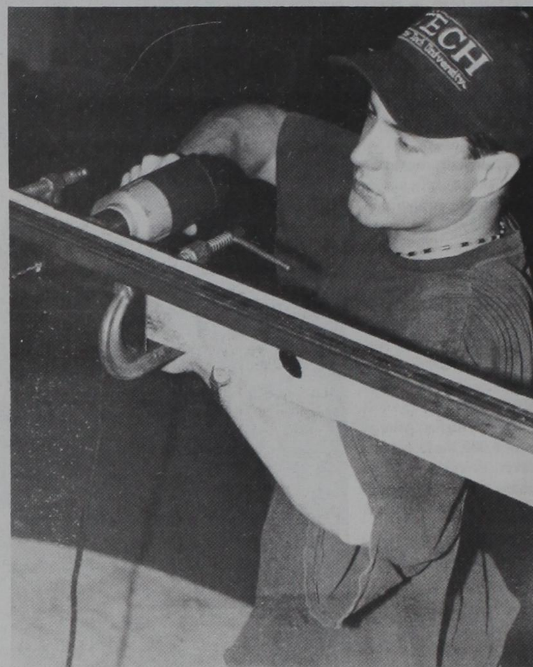
Matt Branum/UD On the scene: Keith Jose, a senior theater arts major from Midland, works on the "Cabaret" set during a theater arts practicum. The set is about 80 percent steel, a new design for Texas Tech University Theatre.
