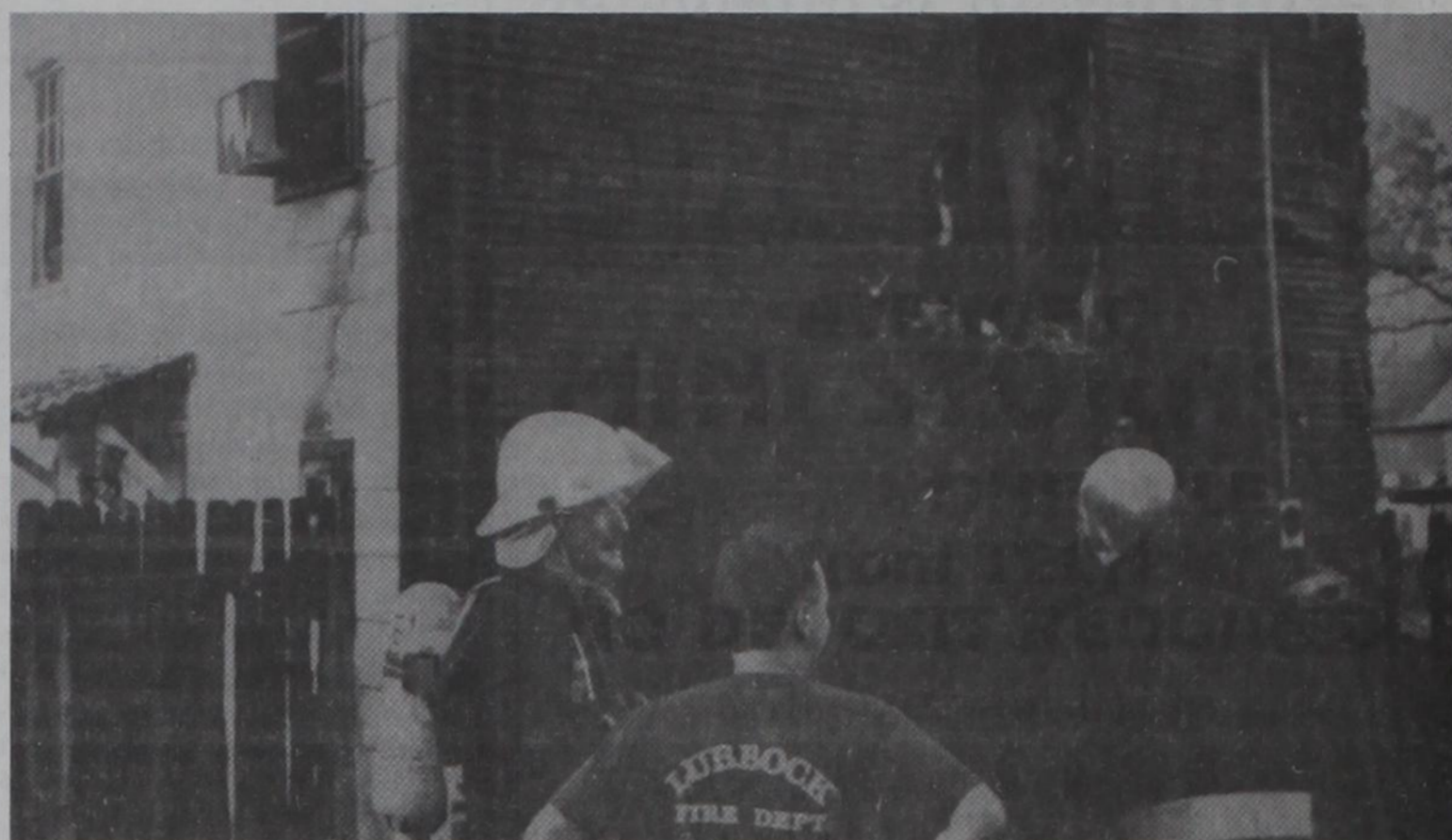
Massive destruction: Members of the Lubbock Fire Department assess the damage Friday night at the destroyed home of Tech student, Kirk Baird, at 2019 16th St. Baird said his only chance of fleeing the burning house was to run through the flames as they engulfed his home. Baird suffered first-degree burns from the fire.
