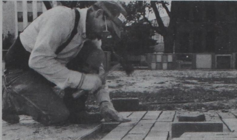
Brick by brick: Martin Cimental, a grounds maintenance employee for 29 years, hammers bricks on the playground behind the human sciences building. The playground will be used by children of different age groups.
