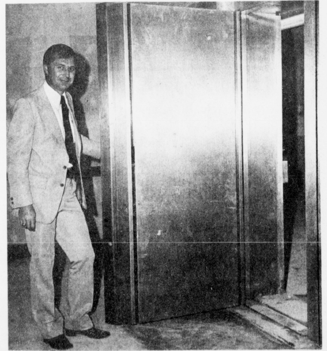
BANK CONSTRUCTION CONTINUES . . . . Construction on the new Muleshoe State Bank building in Muleshoe is continuing on schedule. Pictured in the new vault of the building is Bob Finney, President Bill Loyd announces that tentative plans are to move into the new facilities on November 10 and 11. An open house has been scheduled at the new bank on Sunday, December 2.
