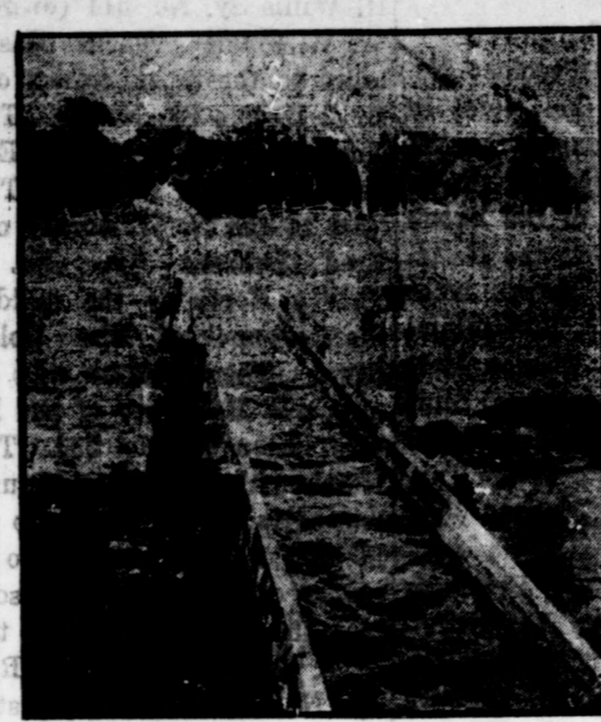
The illustration shows a modern flume constructed of sheet iron three feet in width and curved to a half circle. This flume is on the farms of J. C. and R. A. Brazil, on the Colorado River in San Saba county. The pumping plant was installed by Hall Machinery Co. of Brownwood and consists of a thirty horsepower Pooos Gasoline Engine and a number six volute pump which will deliver 1200 gallons of water per minute at an elevation of 58 feet above the water level in the river. The plant is an unusually efficient one and is large enough to water 125 acres at a cost of thirty-five cents for fuel for each three-inch wetting on an acre of land.
