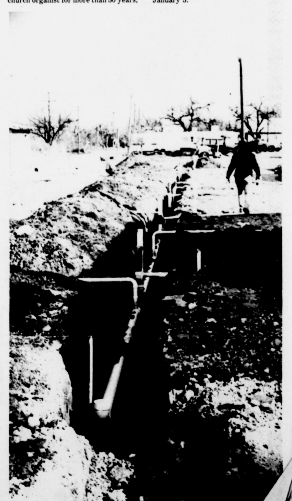
GROUND WORK—Workmen last week started work installing some of the pipes for the new twelve-unit apartment project being constructed in
