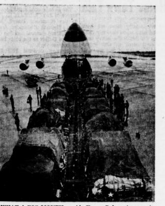
WHAT A BIG MOUTH an Air Force Galaxy transport has, the better to swallow up a consignment of covered howitzers and 1<sup>1</sup>/<sub>4</sub>-ton trucks. Looking like a hungry shark, the huge plane opens up to receive air drop cargo during a readiness exercise at Hunter Army Airfield Ga.
