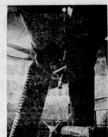
SPACE-SUITED GIANT? What appear to be legs of a space-suited giant are really huge ducts that recirculate air in a room used for testing air conditioners.
