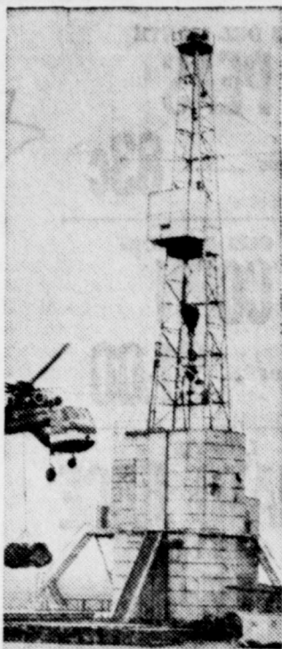
MOVING DAY in Alaska's far north calls for special equipment. Helicopter ferries drilling rig parts from one site to another across the frozen tundra.
