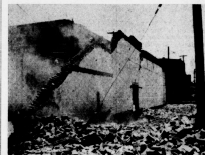
GOING . . . Part of the wall of the old Stoll Building on West Dale Street collapses as a cable fastened around the wall and to a winch on a truck is tightened. The building is being torn down to make room for a parking lot for The Winters State Bank.
