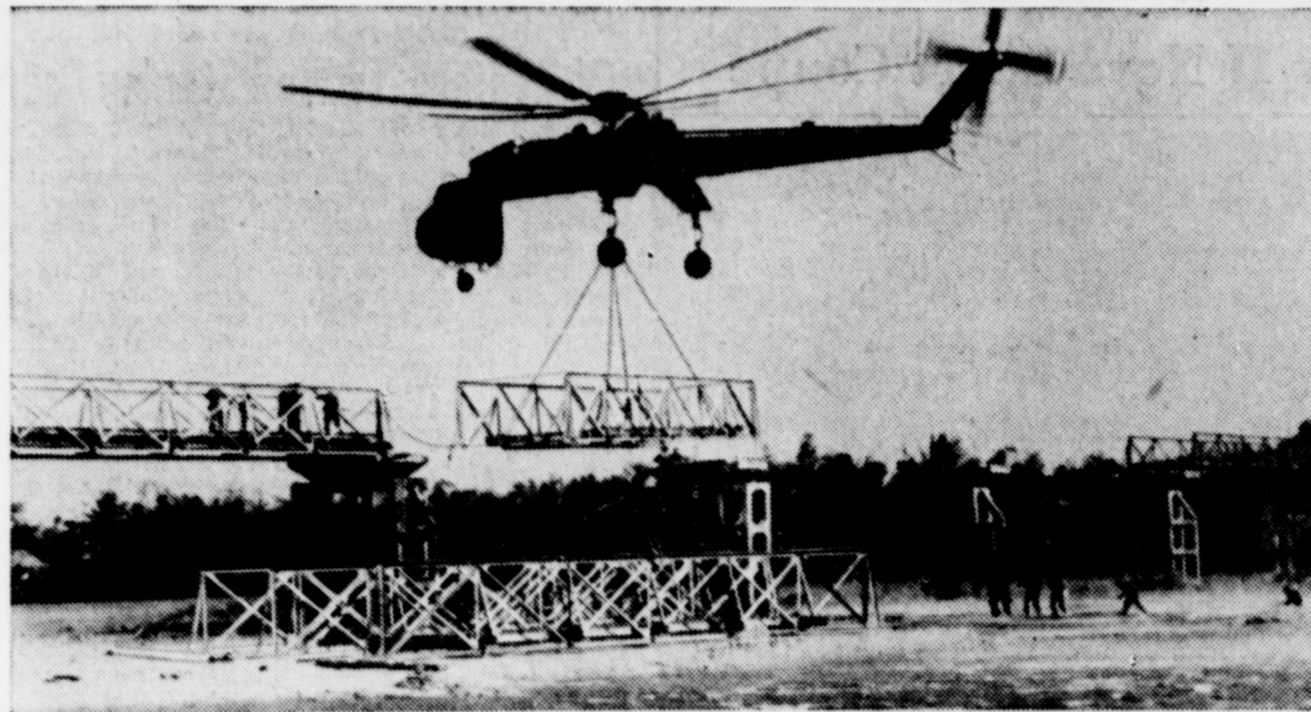
'FLYING CRANE' saves thousands of man-hours in valuable construction time in Vietnam. Here the CH-54 places an 18,000-pound bridge span on pillars for a structure across a South Vietnamese river.
