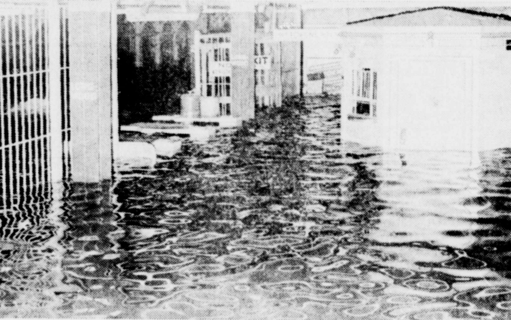
DEEP QUESTION —The Longwood Avenue station of the Pelham Bay subway line looked more like New York harbor when this picture was taken. A busted main flooded the station with four feet of water and caused emergency crews to work around the clock in an effort to restore service.
