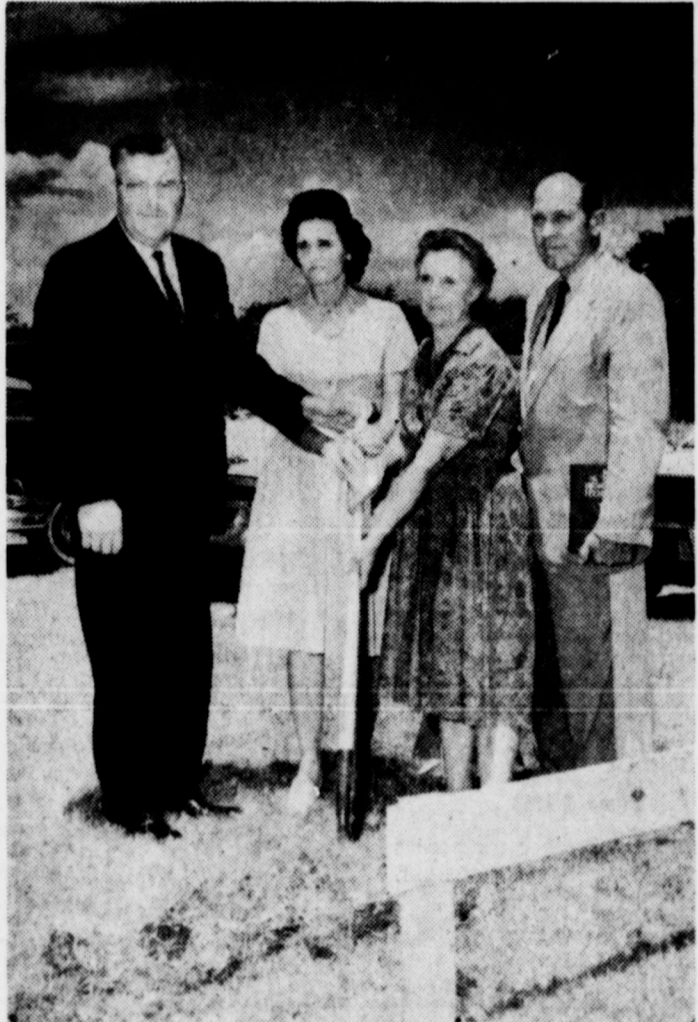
GROUND BREAKING — The pastor and three charter members of the Southside Baptist Church break ground for construction of the new auditorium which is being held. Ground-breaking exercises were held Sunday noon following the regular Sunday church services.
