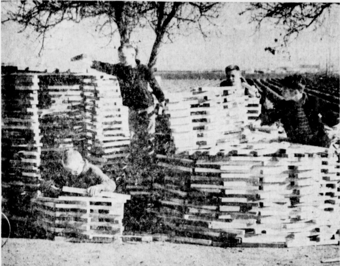
FRAGILE CASTLE —There isn't a single nail in this dwelling. Using some 5,000 pieces of scrap lumber from a nearby mill, these four Watsonville, Calif., boys erected a fragile wooden castle. It has three rooms so far, but there will be more.
