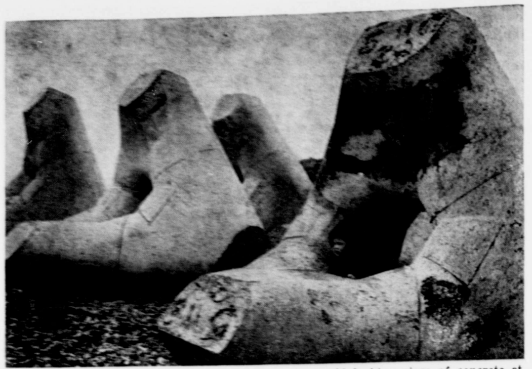
TONS OF FUN—Nigel Sayers, 8 peers out from an odd looking piece of concrete at Shoreham-on-Sea, England. Called stabots, they interlock and are used to form a slope to guard the beachfront against the battering sea. Nigel appears to think that they make fine playthings, even if they do weigh seven tons each.
