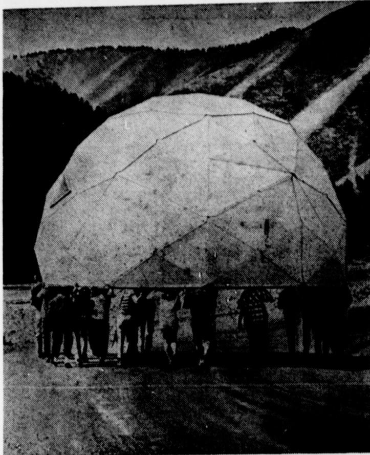
HOUSE-MOVING PARTY — John Koppes, of Sun Valley, Idaho, and some friends move his dome shelter to a local ski run. They carried the lightweight dome shelter about two miles.
