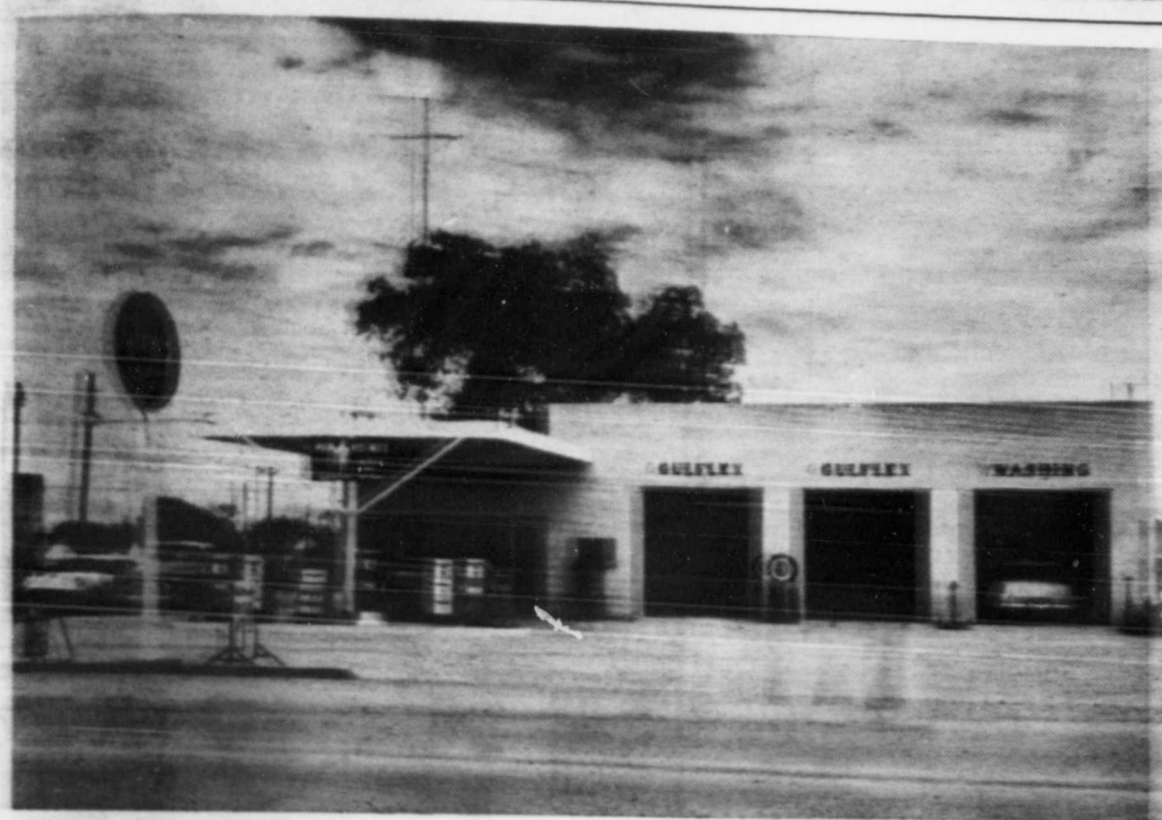
NEW STATION — Roy E. Young will host a Grand Opening celebration at his new Gulf Service Station on North Main St. Friday and Saturday. The recently completed station offers wide driveways, two enclosed lift bays, and enclosed wash bay, and large sales room. (Photo by Little)
