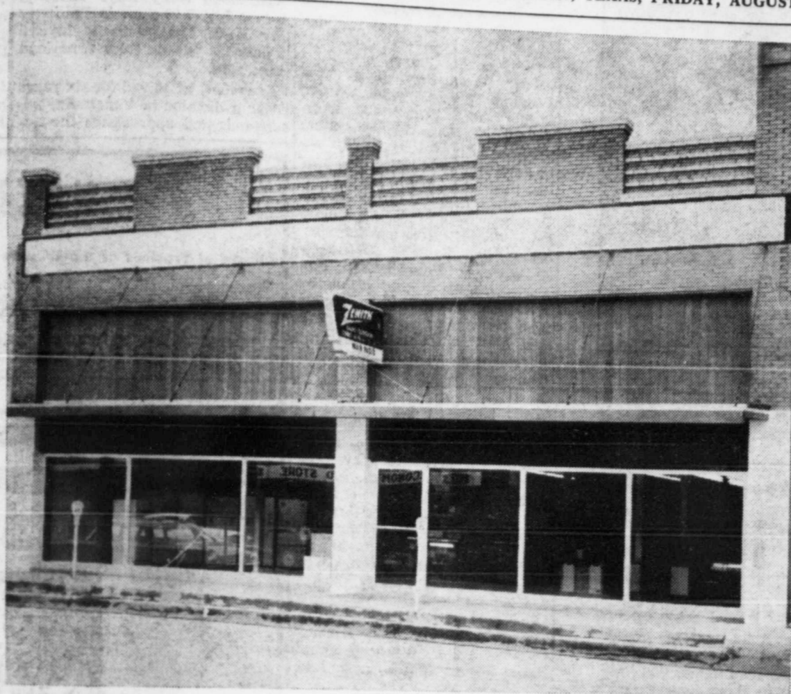
MODERN QUARTERS: A brand new front, remodeled and redecorated interior, and an expansive showroom area are featured in the new home of Main Radio-TV on West Dale. The new home of the old established Winters business offers much more room for display of merchandise. A Grand Opening and open house are planned for today (Friday) from 2 until 5 o'clock. (Little Photo)
