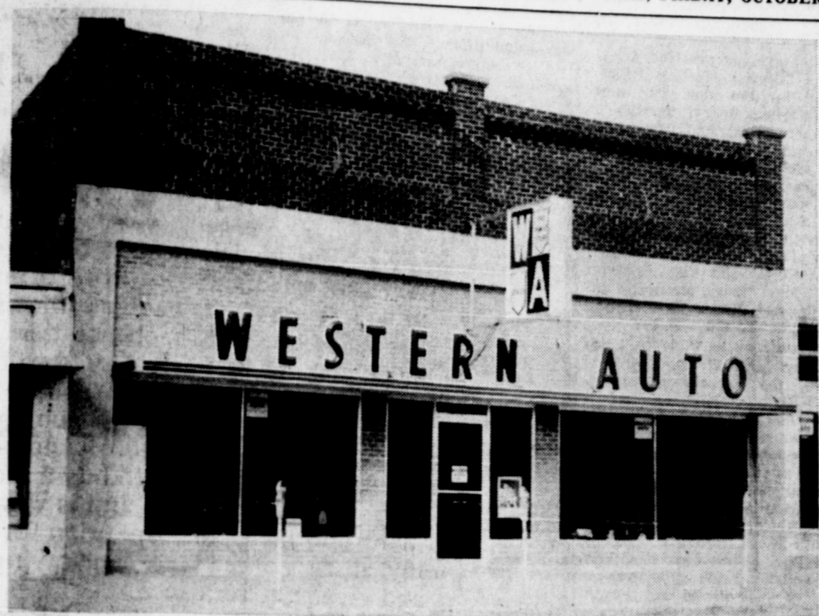
NEW QUARTERS — Above is shown the remodeled building at 135 North Main now occupied by Western Auto. The business is owned by Mr. and Mrs. W. M. Hays, who recently moved the store from their old location one door north. They will hold their open house in the newly remodeled and redecorated and spacious store Saturday, October 14. (Photo by Little)
