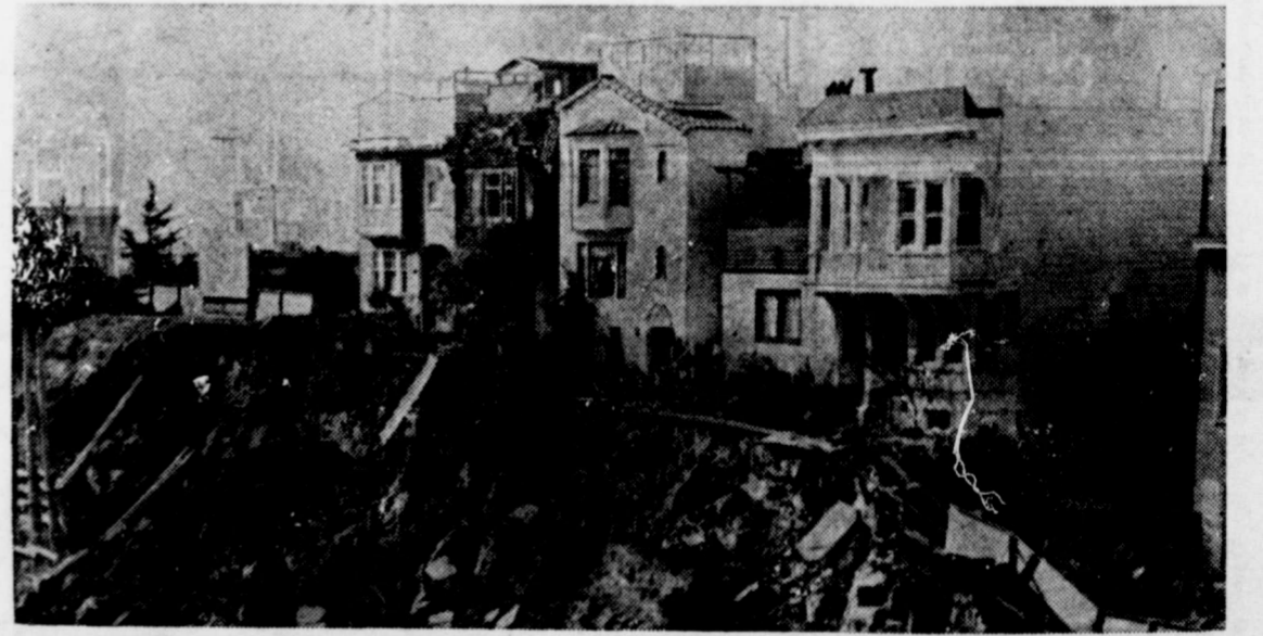
CLIFF DWELLERS —Residents of five San Francisco, Calif., apartment houses were evacuated after a landslide into the site of a 16-story building.
