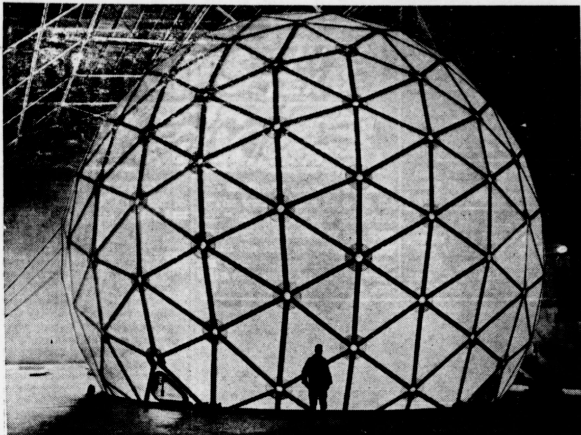
GIANT'S "EYE" GLASSES —Man, lower center, is dwarfed to insignificance by the world's largest glass fiber radome. The huge shelter for a radar antenna is 68 feet in diameter and more than seven stories tall. Laminated plastic panels bolted together in a few basic panel groups can be erected or disassembled in about 80 hours by a six-man crew. The unit, shown in a hanger in Akron, Ohio, weighs some 30,000 pounds, all told. It takes up shipping space the equivalent of eight boxcars, but units are so light that they can be airlifted. The forerunner of radomes well over 100 feet in diameter, it was built for the Air Force.
