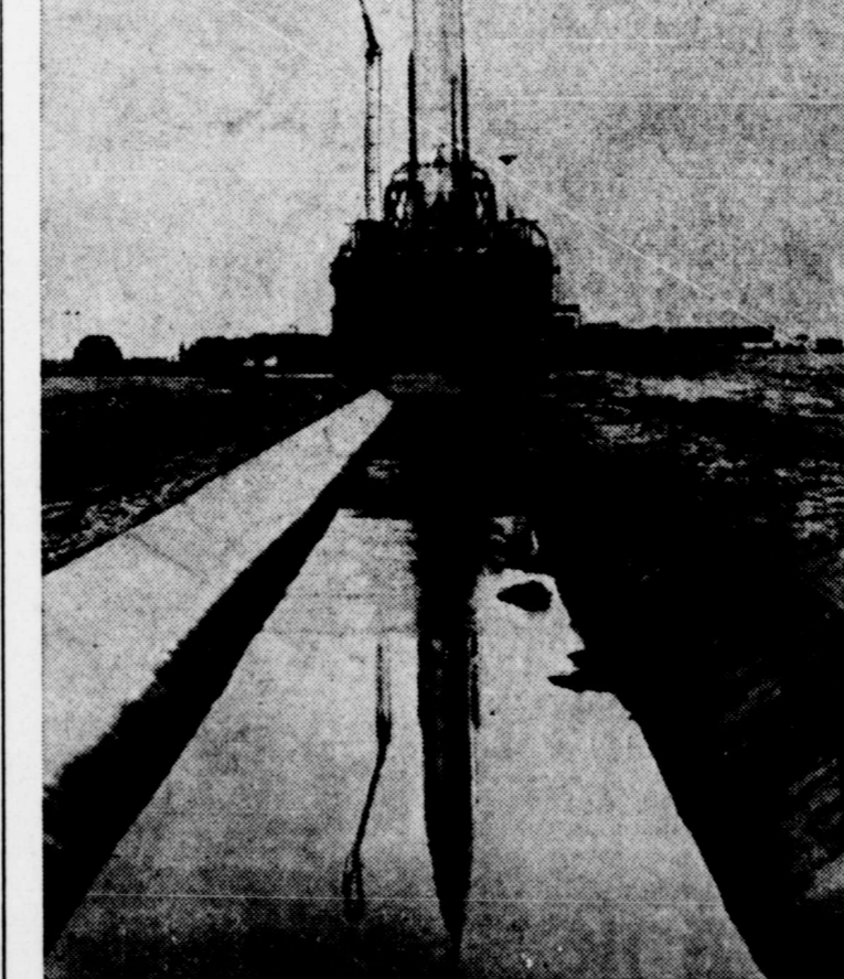
MIRRORING THE FUTURE — The Atlas missile which became the world's first "talking" satellite is shown, above, in an unusual mirror-pool shot on the launching pad at Cape Canaveral, Fla. Water trough is part of the system that takes care of tremendous heat generated at blast-off.
