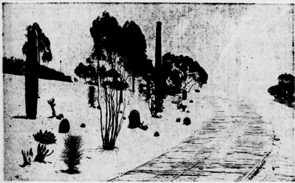
The original Yuma Road, which with eight other famous trails of the Southwest, will be reproduced for visitors to the Ford Exposition opening in Dallas, June 6, stretches across the desert between El Centro, California, and Yuma, Arizona. It is part of the old Spanish Trail from Florida to California. About 20 years ago planks were laid on the shifting sands of the desert, to wind their way like a writhing snake across the dunes.
