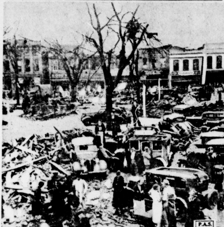
ATLANTA . . . Here is shown but one of the storm strewn scenes which Georgians and other Southern state citizens faced when the most destructive tornado in years had taken its toll of nearly 500 lives and damaged property, estimated into millions. This photo shows a portion of the business section at Gainesville after the tornado had passed and the job of rebuilding started.
