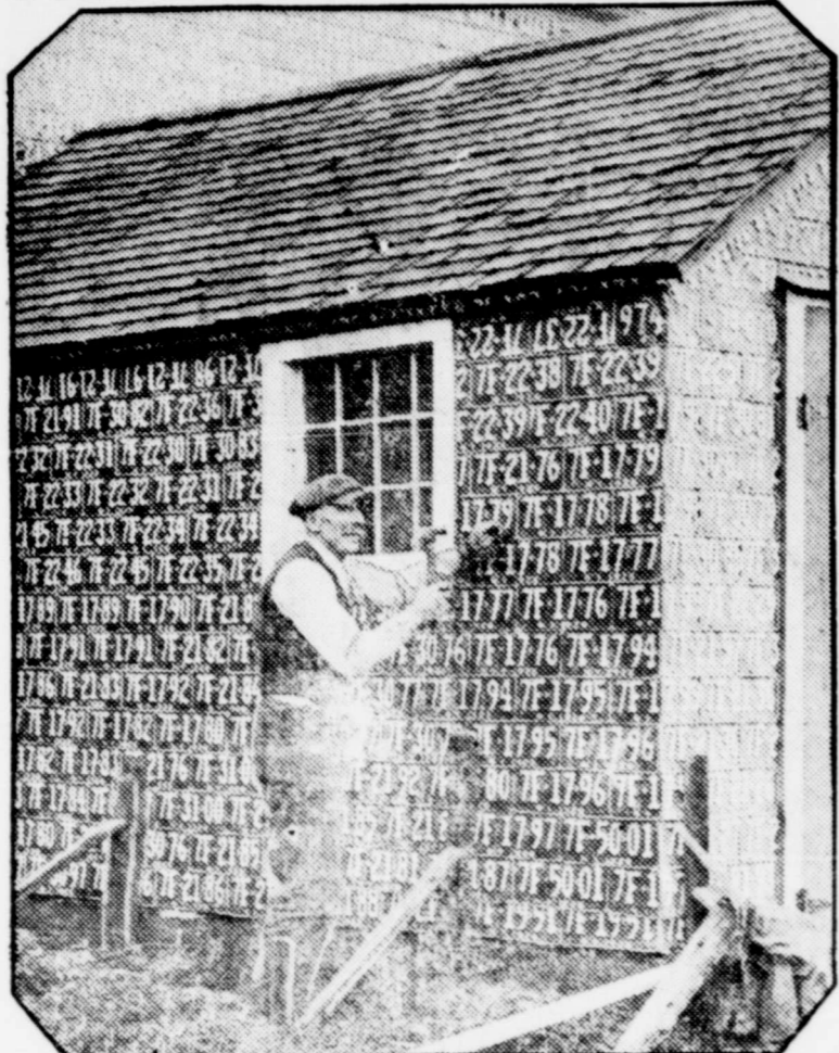
It would be pretty hard to "get the number" of Albert H. Libby, a farmer of near Forestville N. Y., because he has nine tons of them. Recently he purchased the unused plates from the county license bureaus and is using them as weather-boarding.
