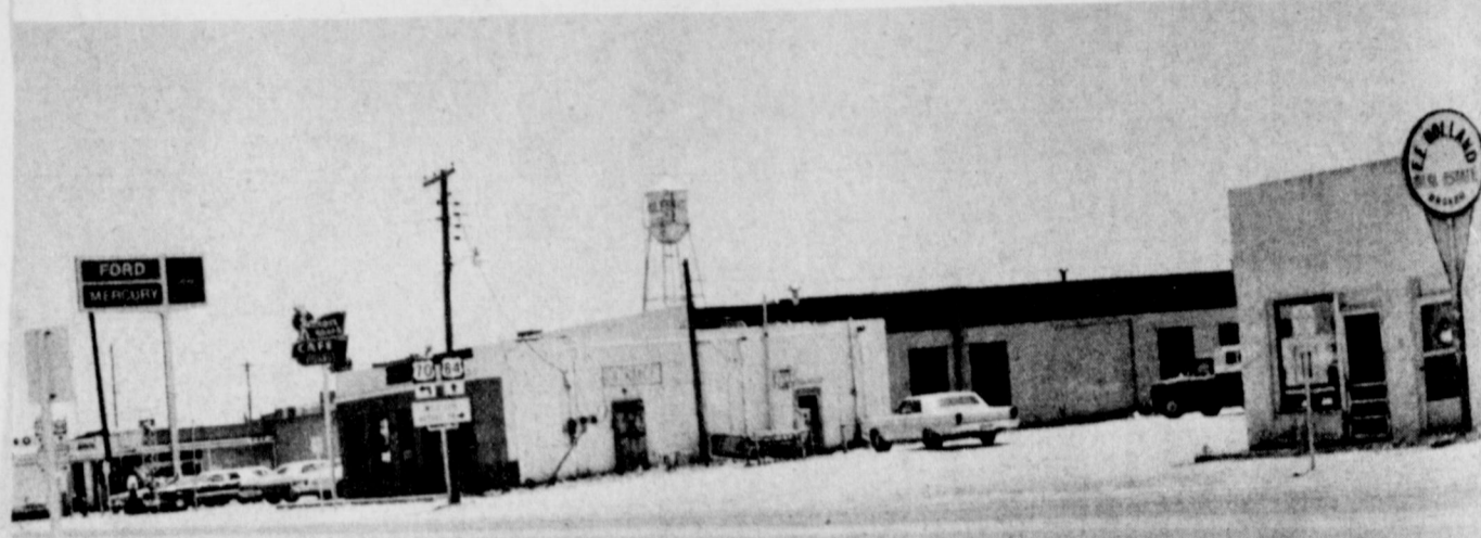
NEW BANK SITE...Muleshoe State Bank has purchased most of the block between American Boulevard and Avenue B and between First and Second Streets for the construction of a new and modern bank building. Construction of the new building is expected to start around the first of the year with completion sometime in the fall of 1973.
