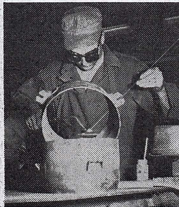
LACING IT UP . . . Pfc. Albert Smith, welder from Palestine, Texas, is shown brazing a bracket on a ball assembly. This type of brazing work is more difficult than ordinary welding. Pfc. Smith was a construction welder before entering army.
