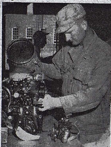
Cpl. Emil Erikson of the Engine Tear-Down department inspects each accessory that is removed from the engines and determines its fitness for further use. Here Cpl. Erikson inspects a carburetor. If it is okay it will be thoroughly cleaned up and put in a used parts pool for use in making repairs.
