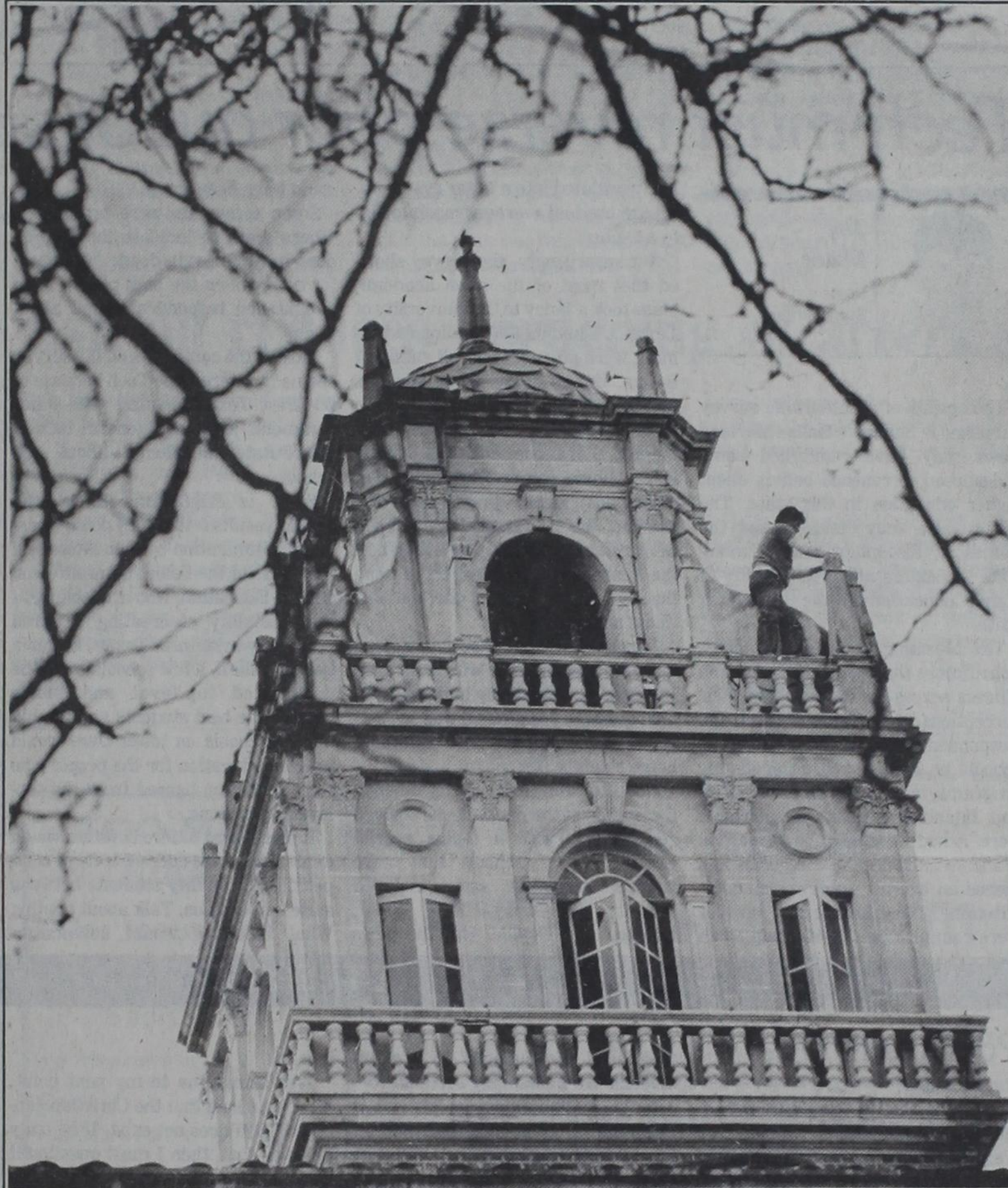
Decking the tower
