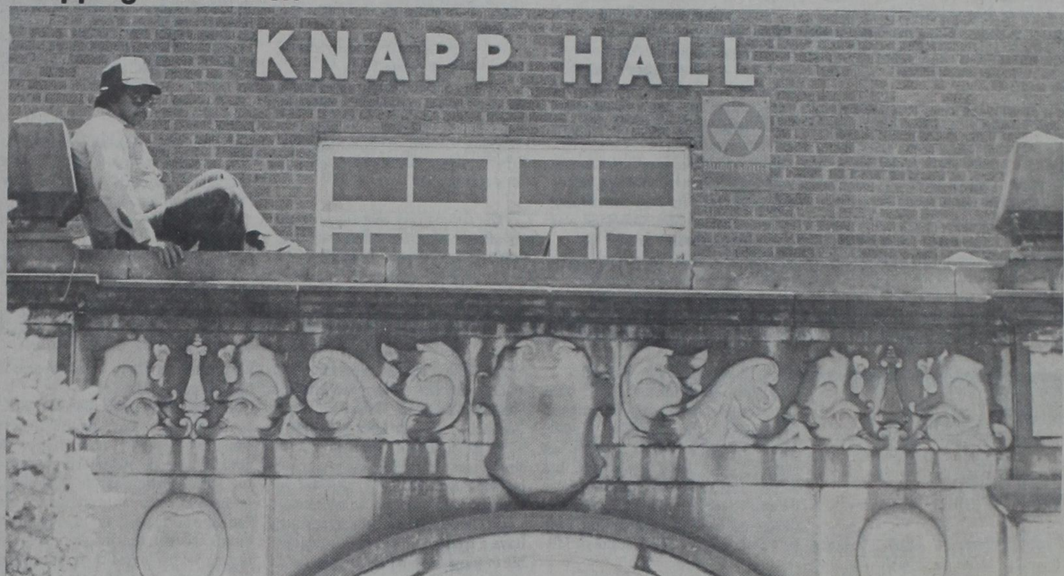
While many were taking their lunch break on the ground, Mickey DeLeon, an employee of Hamilton Roofing of Lubbock, has a good view of the campus from the roof of Knapp Hall, where he took a break during the lunch hour Wednesday.
