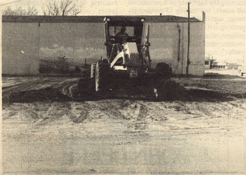
DAMAGED BY FIRE in 1947, then partially rebuilt, Plains Frozen Foods, owned and operated from 1946 until 1963 by Dick McGinty, the building has now been razed and the lot leveled and cleaned.
