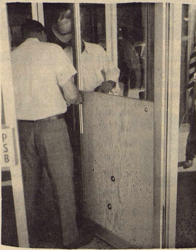
Wood panel covers broken glass in Bank door.
