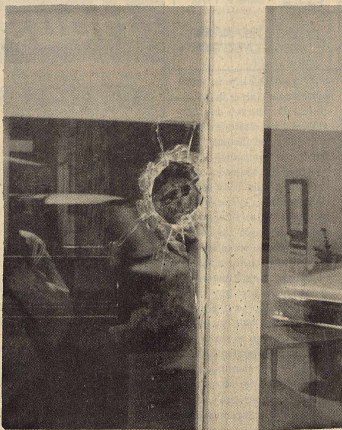
Hole in east Bank window.
