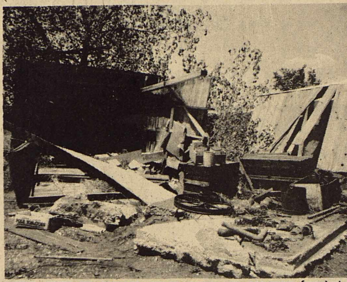
Break stunt by twister which ripped up concrete foundation but left trunks with paint cans on top.
