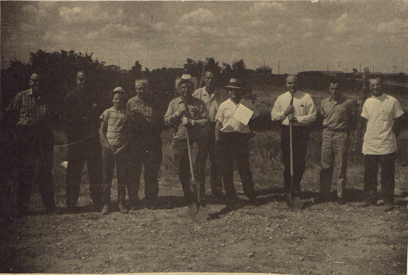
GROUND BREAKING---The group pictured above took part in the formal ground breaking ceremony for the new convalescent home which is to be built here very soon. They are, left to right, Melvin Smith, the promoter; W. A. Crowder, the masonry contractor; Alton McGinty, son of
