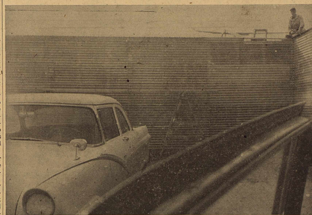
CURRENTLY UNDER CONSTRUCTION is a 30 by 40 foot addition to the garage section of the Plains Motor Company. Shown "on the job" is Newt Rowland, who with Pete Smith are constructing the addition. According to
