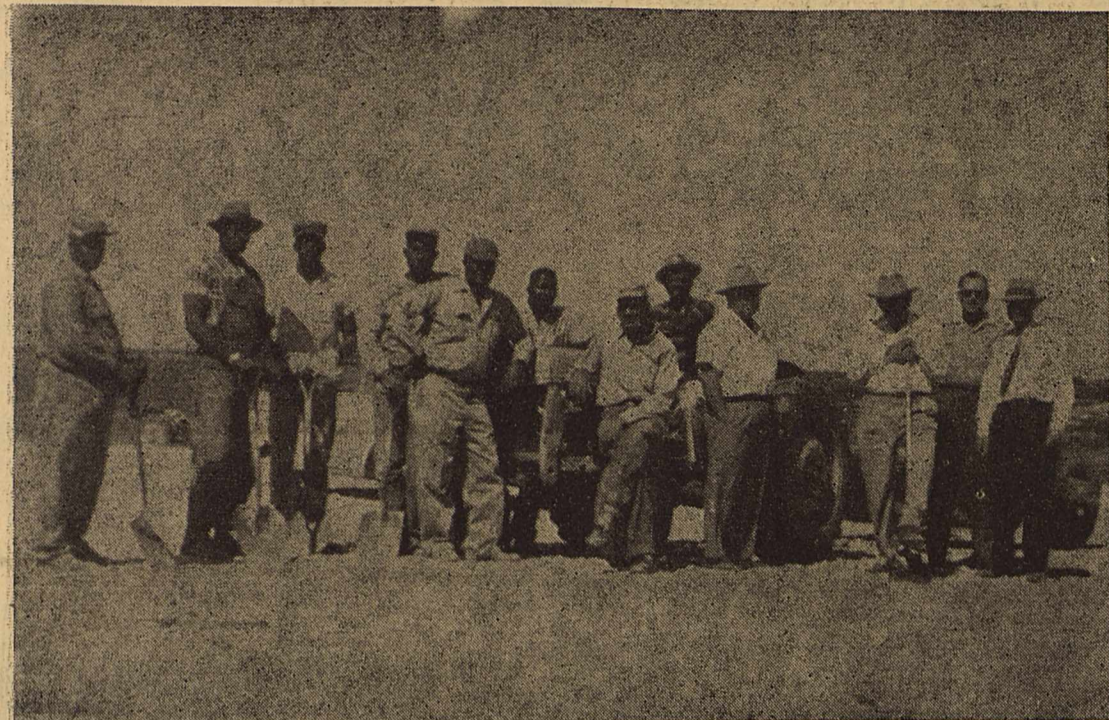
WORK ON THE NEW COTTON WAREHOUSE to serve the surrounding areas got underway Monday. Shown here with a group of the workmen are at left, F. Z. Payne of
