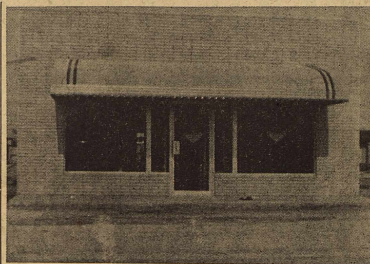
NEARLY COMPLETE is the Curry Building, just east of the courthouse, which will open in about three weeks as a variety and drug store. The modern brick structure, built by Mr. and Mrs. Joe Curry, is one of which they may well be proud, as well as being an asset to the entire town. REVIEW Photo
