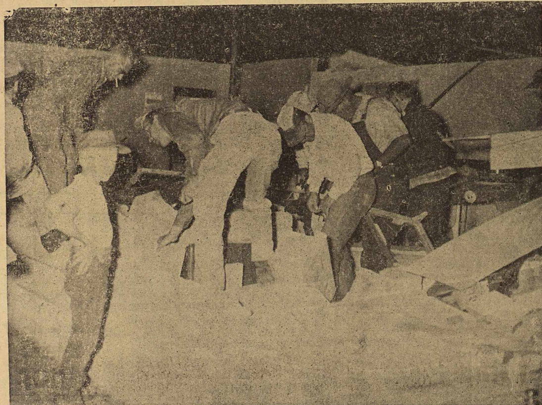
VOLUNTEER WORKERS plunged in with a will Wednesday night to salvage what equipment they could at the Been Laundry, which was almost demolished by the tornado.
