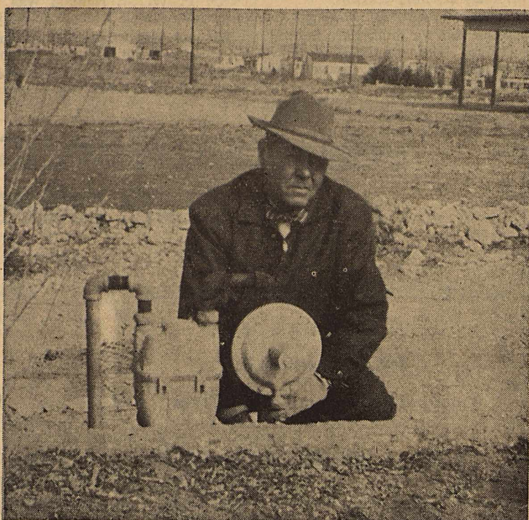
Bill Ashenbeck is seen above as he turns on gas meters around town Tuesday morning after the main gas line was broken and service off for three hours.
