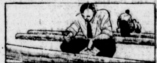
Testing for decay with a pole prod
