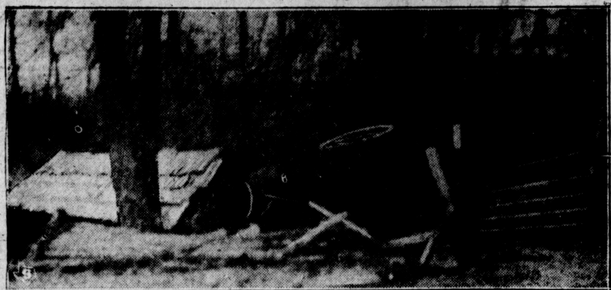
Here is all that is left of the residence of L. L. McKikel, seven miles south of Detroit, Texas, after a disastrous tornado swept through North East Texas. Although house, barns and outhouses were completely demolished, the McKikel family was unhurt. Thirty were injured in the 45-mile path of the twister, however, and two were killed. This photo was taken in the rain.
