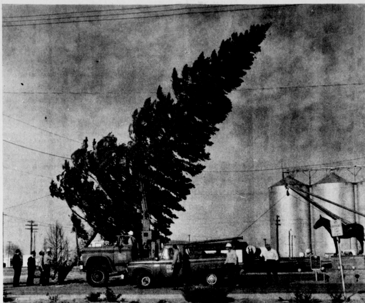
INTO PLACE --- This towering tree, brought down from the mountains near Cloudcroft, N. M., is shown being lifted into an upright position by Bailey County Electric Cooperative trucks and employees. The tree was anchored and decorated for the Christmas holiday season. Pictured around the tree are John Shelton, Harvey Bass, Harold Cowan, Clovis Windham, Ray Terrell, Jim Shafer, Seth Shaw and Grady Edelman. Cowan, Windham, Terrell, Shafer and Shaw are employees of Bailey County Electric. Those going to Cloudcroft to bring back the tree were John Shelton, Harvey Bass, Lindell Murray, Alan Burrows and Harold Cowan. King Brothers provided a truck for hauling the tree back.
