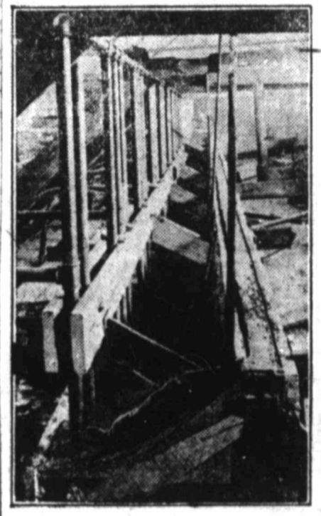
FIG. XVI.—MAKING CEMENT MANGERS.
