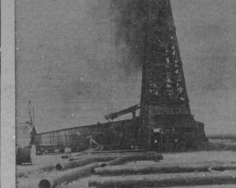
SANTA RITA, 1923 — This well drilled on University of Texas land in West Texas opened up the Big Lake field, May 28, 1923, from a depth of 3,028 feet, and drew attention to the now famous Permian Basin oil province and put the first "oil money" in the University Permanent Fund, which now holds more than $447 million from royalties, rentals and bonuses.
