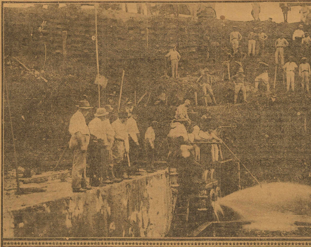
Before the Gamboa dike in the Panama canal was blown up a considerable amount of water was let into the Culebra cut through pipes in the dike. Our photograph shows the first opening of the valves of these pipes, in the presence of Colonel Goethals and other officials.
