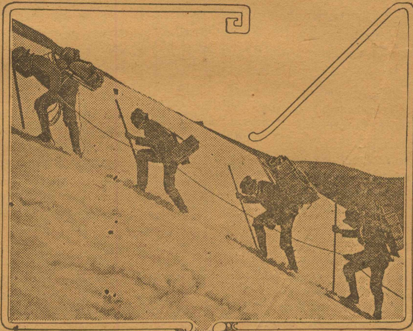
SURVEYORS CLIMBING MOUNTAIN
