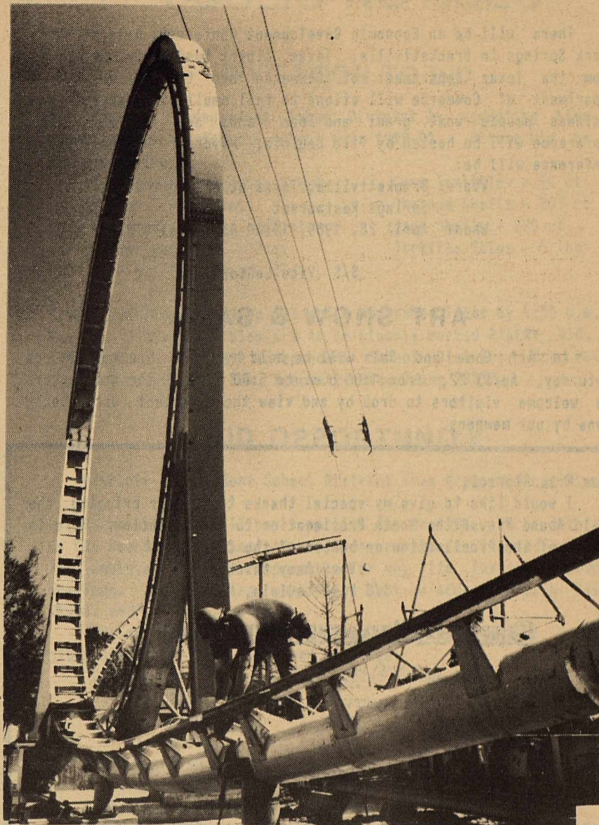
HOUSTON, TEXAS...Coaster enthusiasts get ready! Construction on the Viper, AstroWorld's new steel loop coaster, nears completion. Workers continue to lay the 1,968 feet of track that will make up the ride. The Viper, which features a 360-degree loop, corkscrew turns and a 60-foot long tunnel, is scheduled to open in late April. AstroWorld, currently open weekends, is a member of the Six Flags family.
